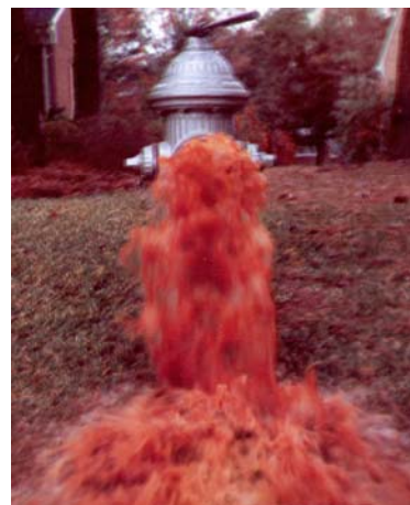
Iron Particles Cause "Red Water"
